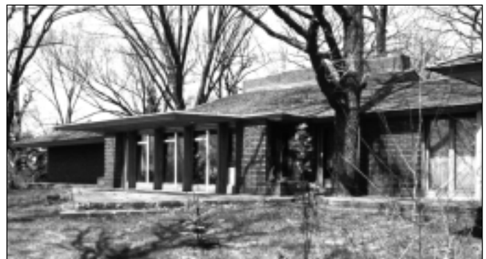
The Willey House in Minneapolis, an example of a Usonian residence. Built in 1934, it is listed on the National Register of Historic Places. The architect was Frank Lloyd Wright.
